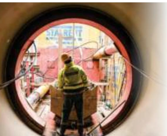
Subor Jacking Pipes are used for the construction and renovation of underground pipelines using trenchless methods.
